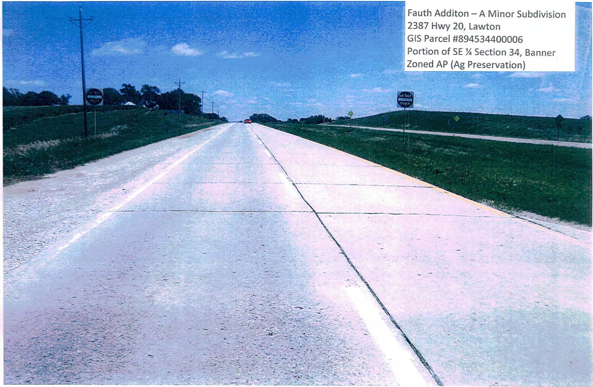
Hwy 20 ROW Looking East from Franklin Ave Intersection
