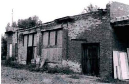
Carpenter Shop before 1998
