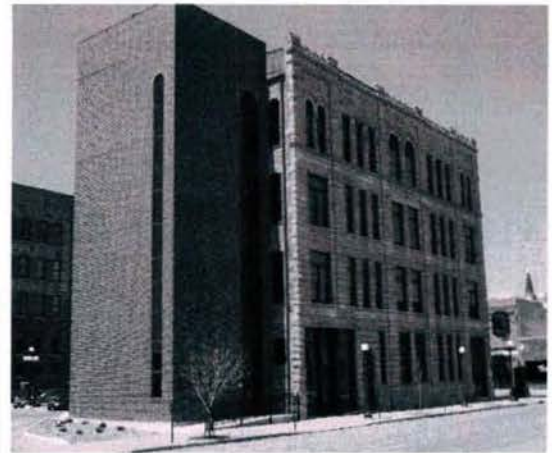
Elevator/Mechanical Tower at South
