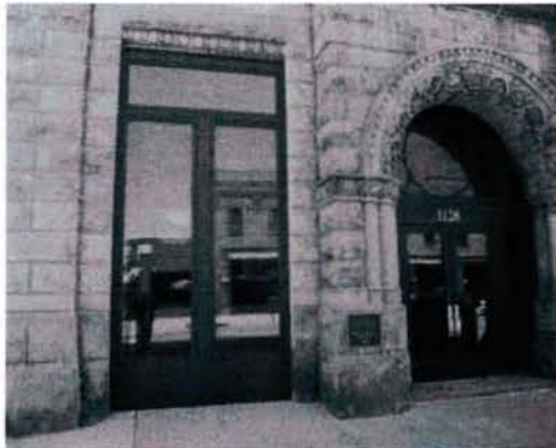
New Windows at North Entrance
