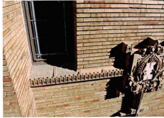
View of Terra Cotta Sill – East of East Masonry Pier
