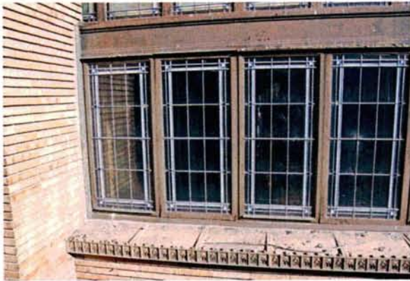
View of Terra Cotta Sill – East End of Center Window
