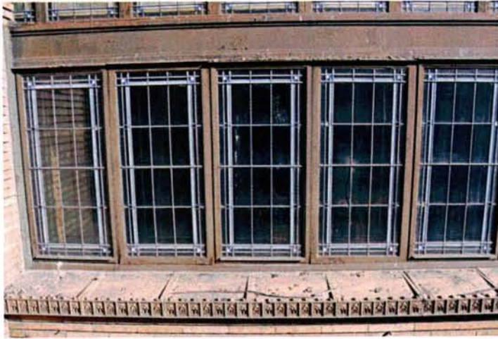
View of West Portion of Center Windows
