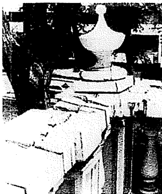
Figure 8. Deterioration of Exposed Detailing. Exposed or freestanding terra-cotta detailing (parapets, urns, balusters, etc.) have traditionally been subject to the most severe vicissitudes of deterioration as a result of freezing temperatures and water. (Colorado State Historic Preservation Office)
