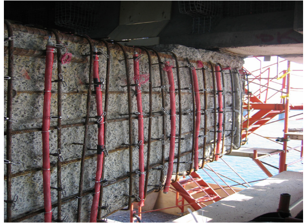
Galvanic anode system on bridge pier prior to concrete placement
