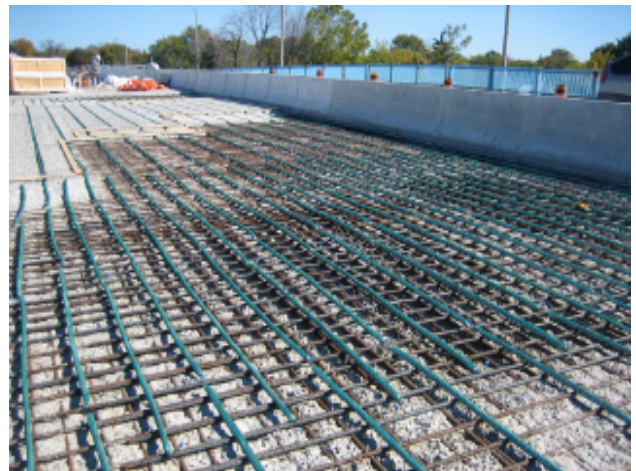
Galvanic anode system on bridge deck prior placement of reinforced concrete overlay
