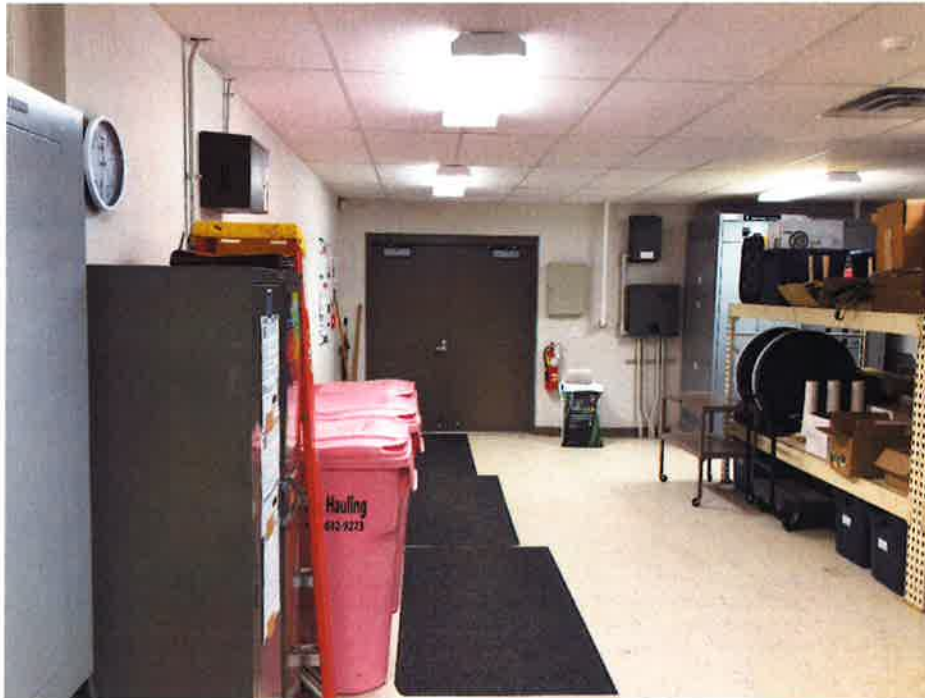
Figure 4.1: A single air diffuser serves the entire employee entrance Rm. 106
