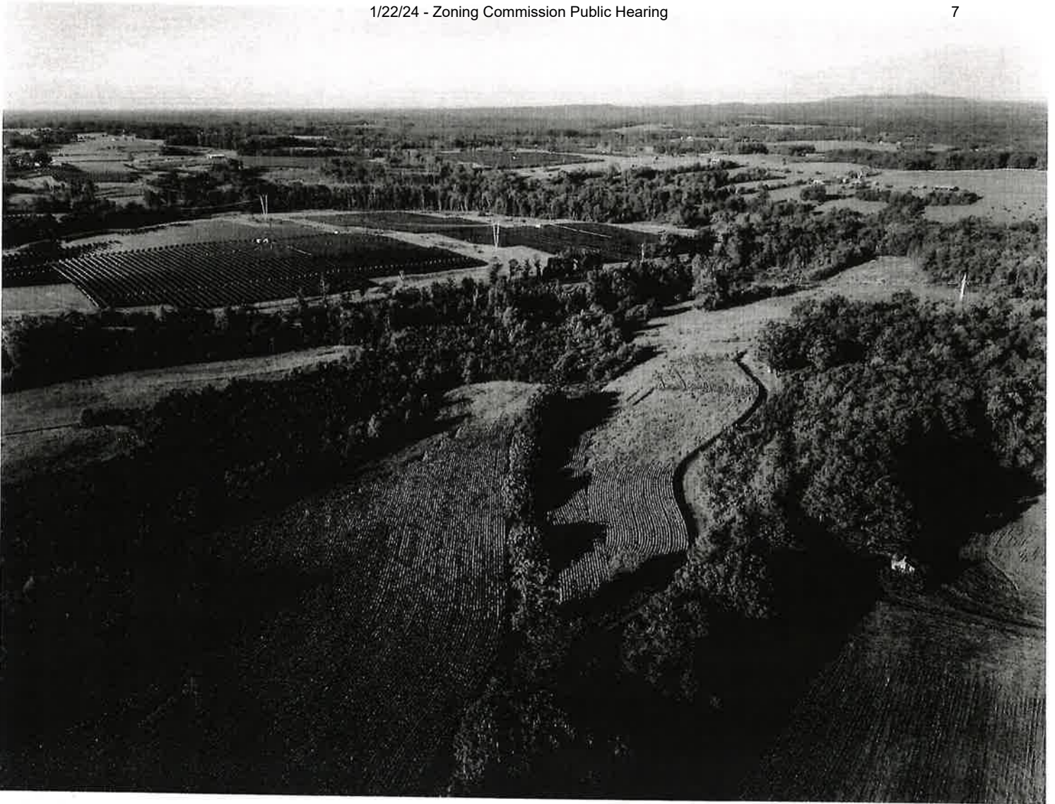
The Amazon Solar Farm, developed by Dominion Energy, in Climax, Va., a 1,500-acre, 120-megawatt project. Melissa Lyttle for The New York Times
