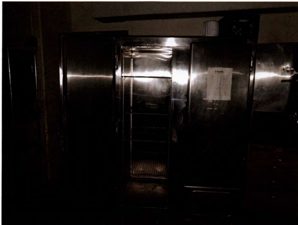
Photograph 8: CFC containing unit (commercial refrigerator)
