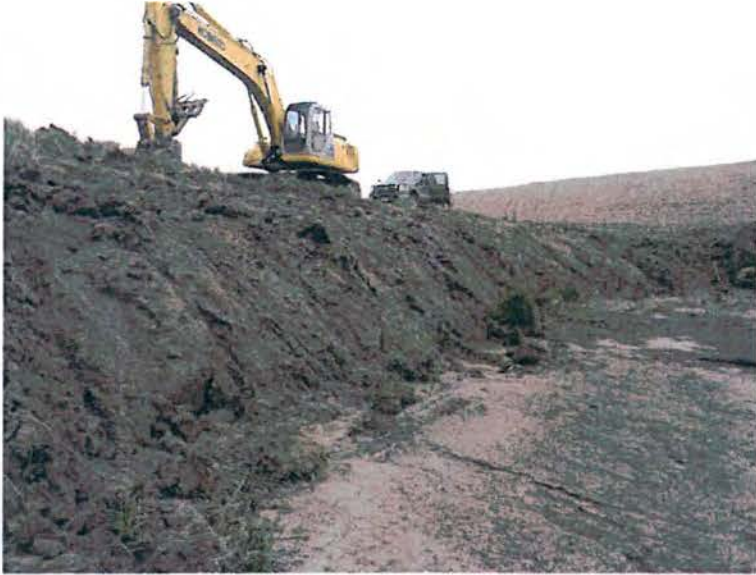
Rebuilt berm and front slope
