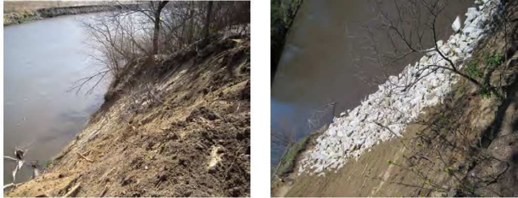
Little Sioux Park Riverbank Armoring Project (Before and After)
