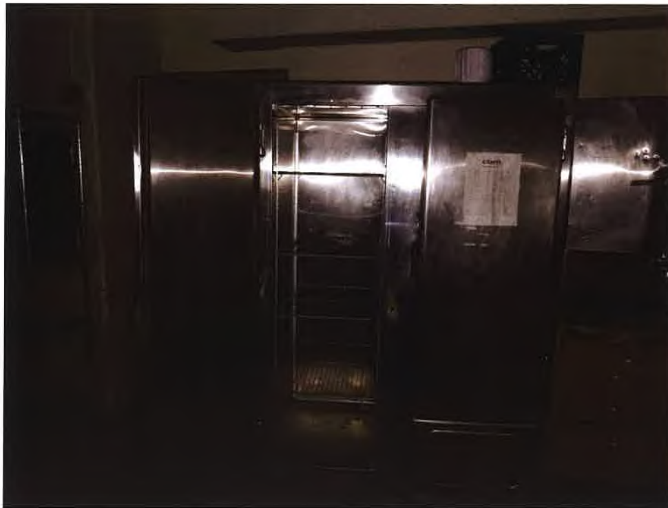
Photograph 8: CFC containing unit (commercial refrigerator)
