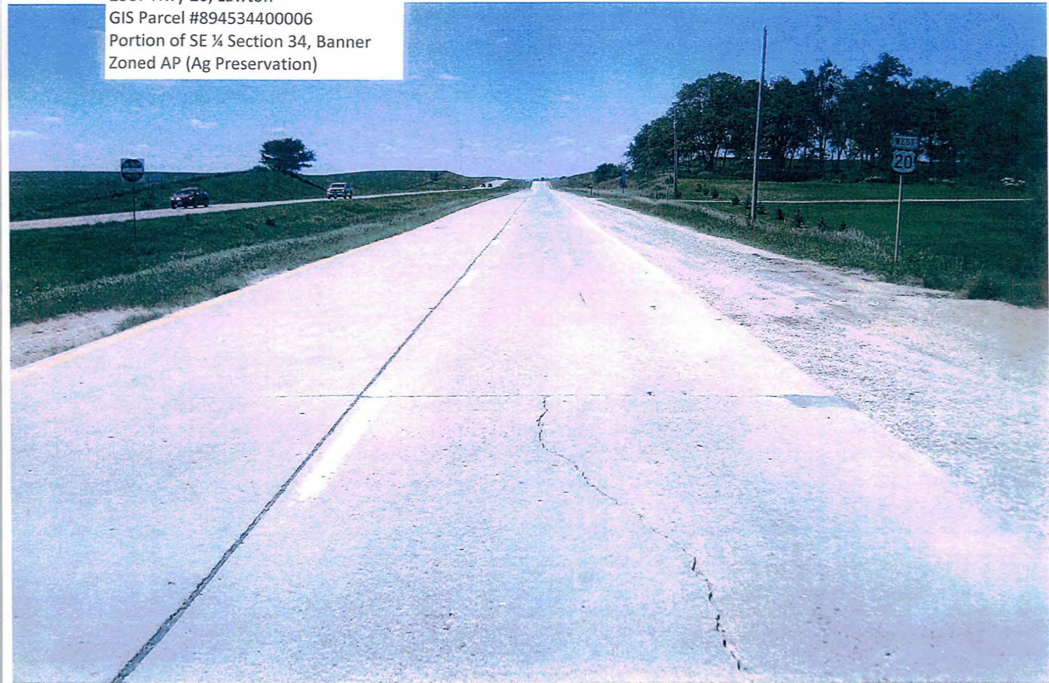
Hwy 20 ROW Looking West from Franklin Ave Intersection
