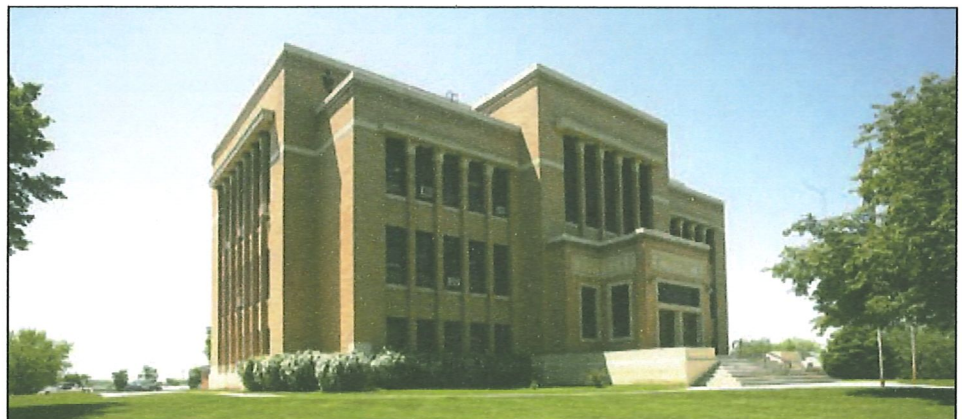
STEELE'S DESIGNS FOR THE 1917 CHARLES MIX COUNTY COURTHOUSE IN SOUTH DAKOTA DREW LIBERALLY FROM THE WOODBURY BUILDING'S STRUCTURE AND DETAILS.
