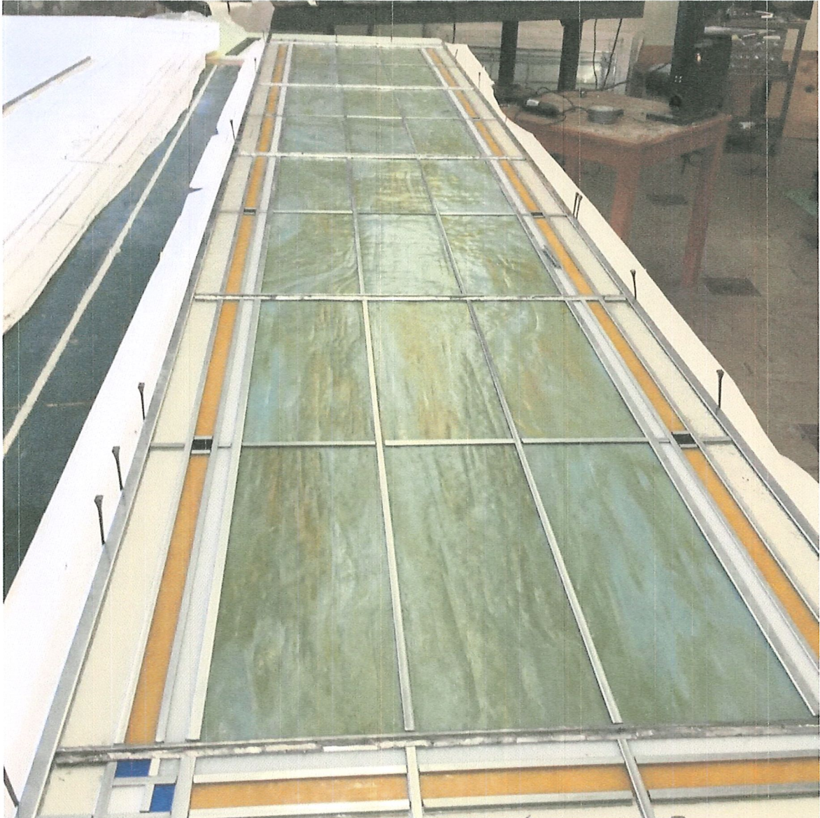
Another window ready for grouting
