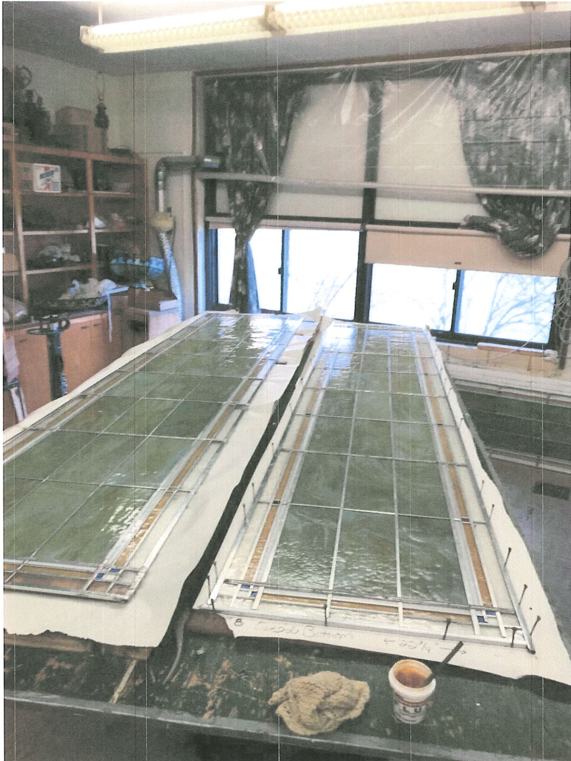
2 windows for Courtroom 207 that have been put back together with new zinc
