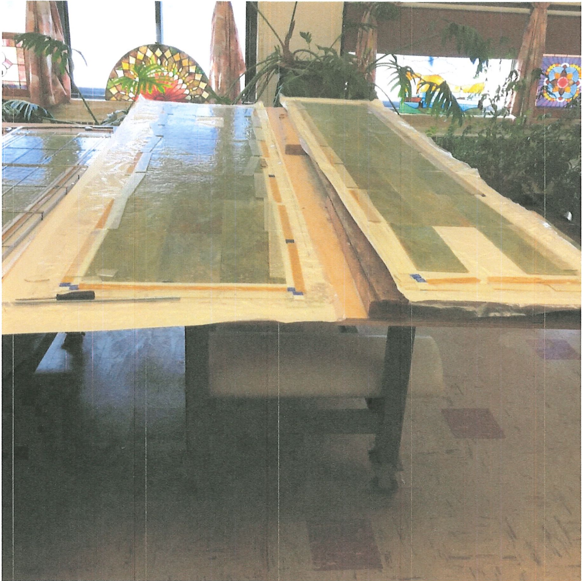
Windows disassembled waiting to be put together
