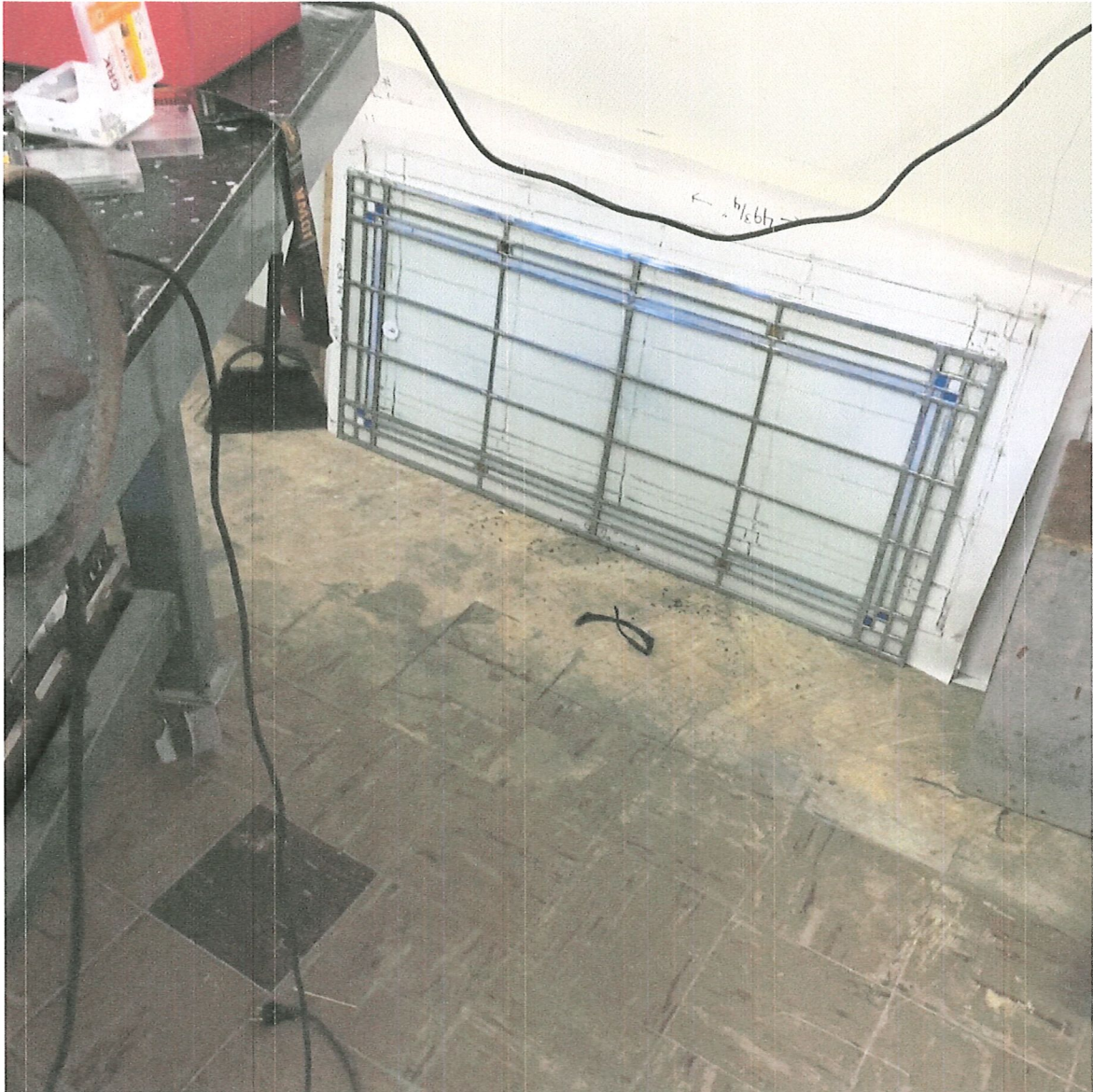
Small windows that are already done
