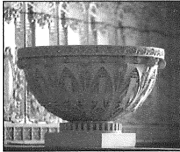
UNDER PURCELL'S DIRECTION, SCULPTOR KRISTIAN SCHNEIDER PREPARED FULL-SCALE MODELS OF ELSMLIE'S ELABORATE INTERIOR DECORATIONS, FROM WHICH TERRA COTTA, IRON AND BRONZE ORNAMENTS WERE CAST.
