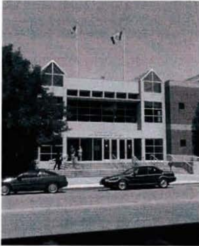
Woodbury County LEC, home of the Jail
