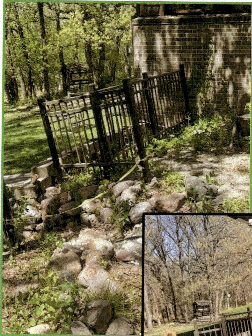
Lower level railing on water feature that are leaning due to shifting soils, this is a liability for us and is an eyesore.
